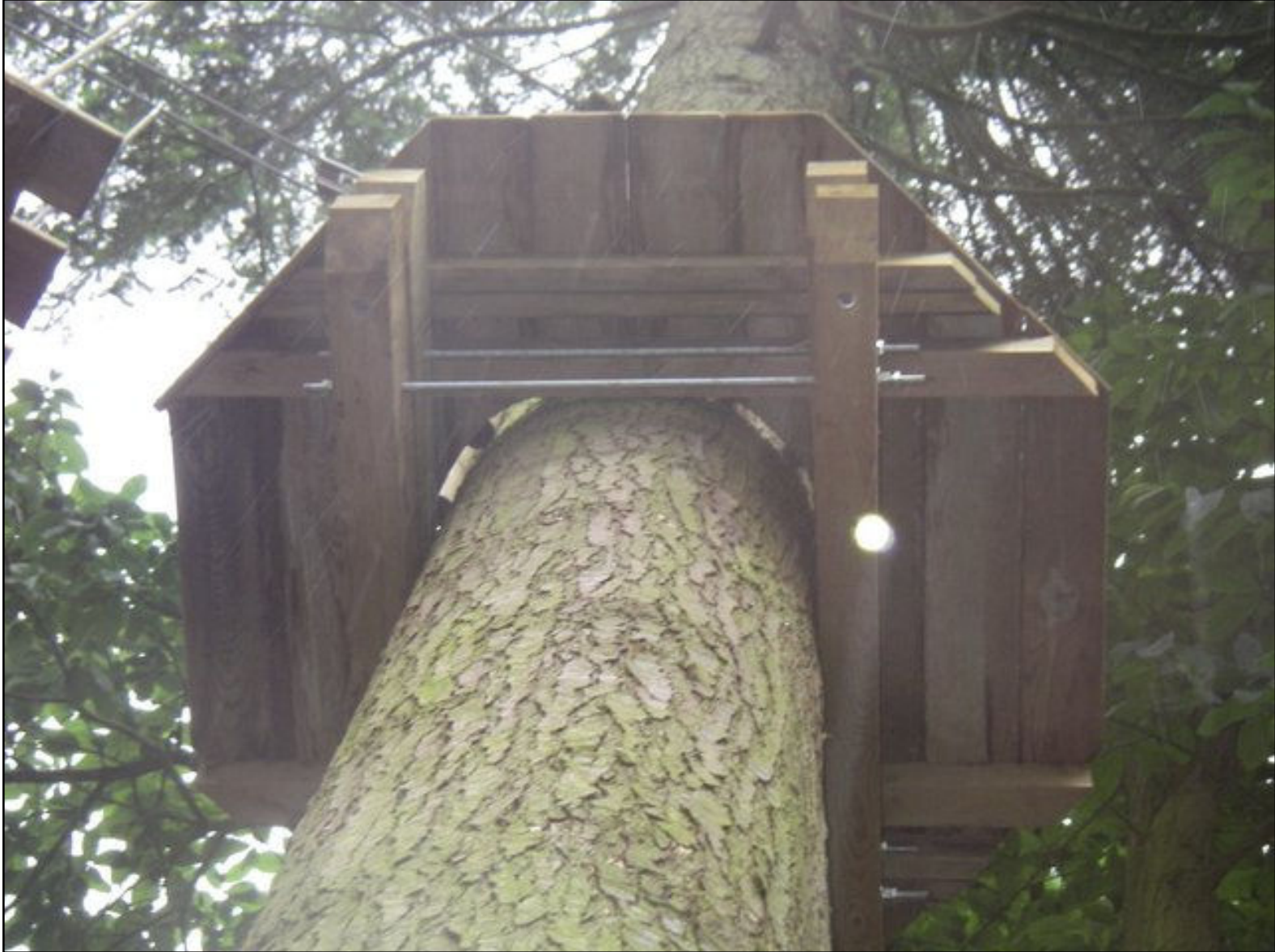
Example of Brace and Platform Construction
